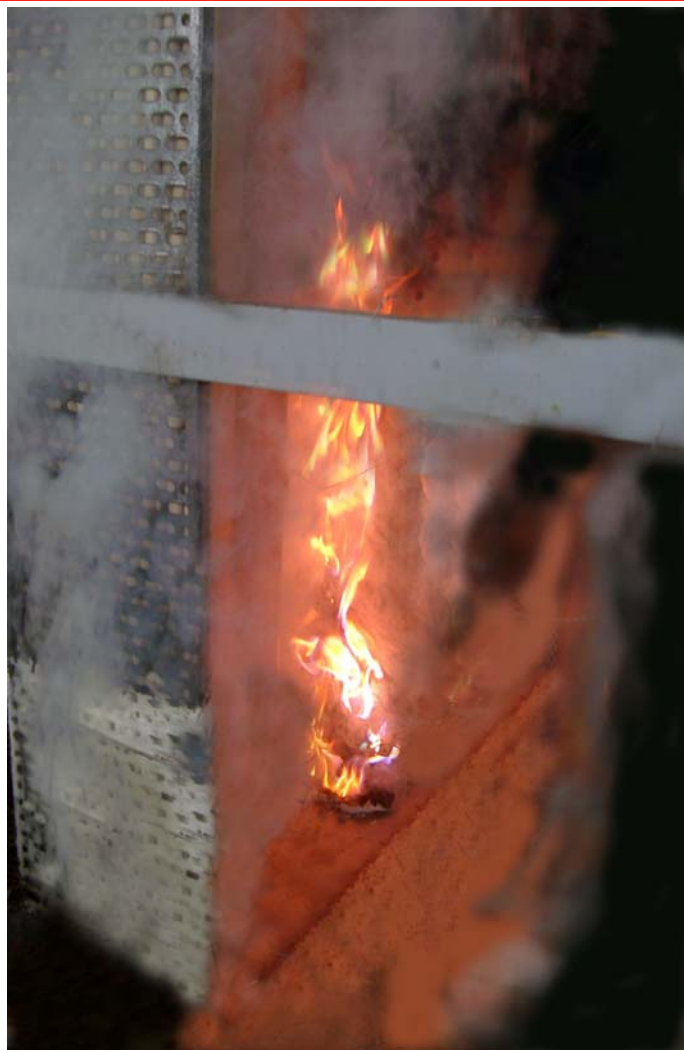
An Unrated Pipe Penetration Fails in a Floor Slab
